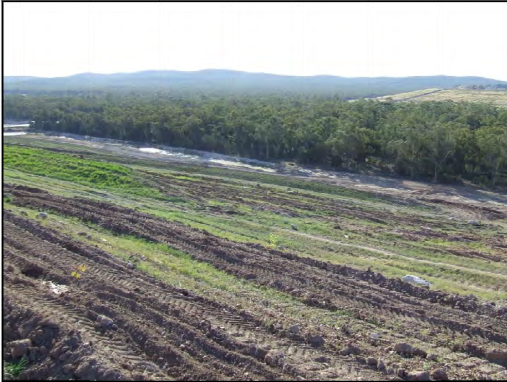
Plate 6 – Rehabilitation at north-west corner of northern emplacement
