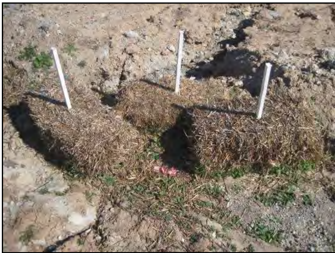
Plate 3 – Hay bales used to control erosion and sedimentation
