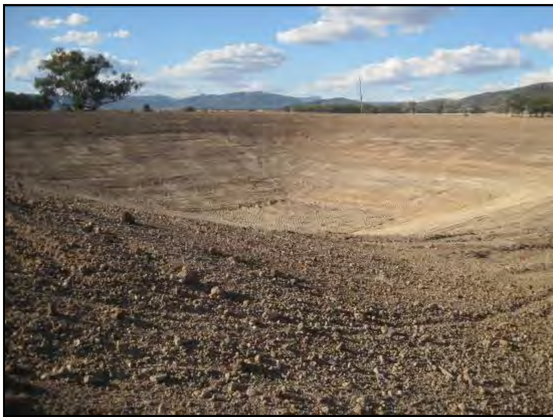
Plate 1 - New Storage Dam North of SB18
