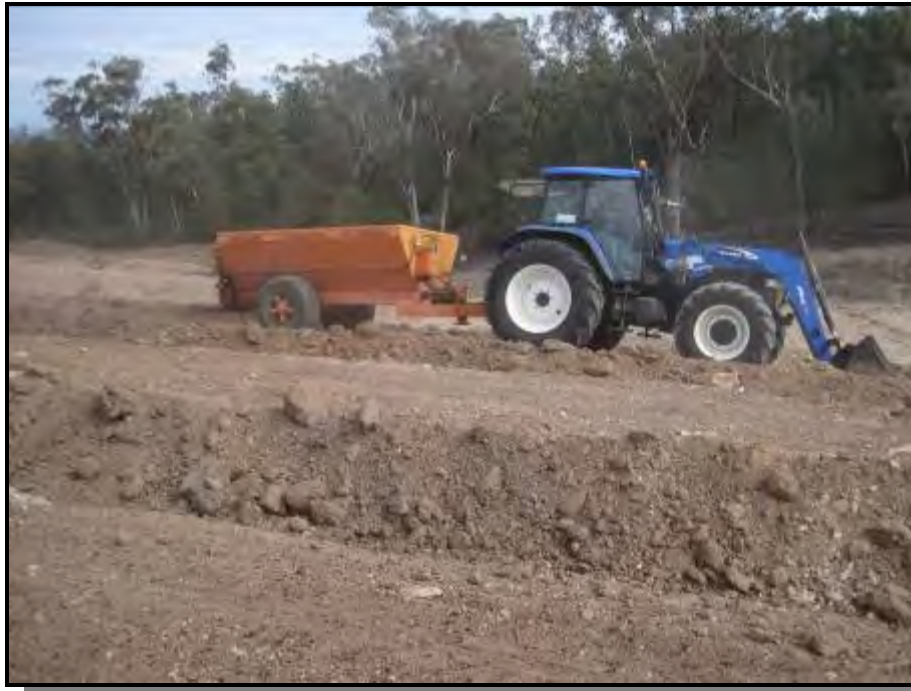
Plate 8 – Applying seed compost mix between tree mounds
