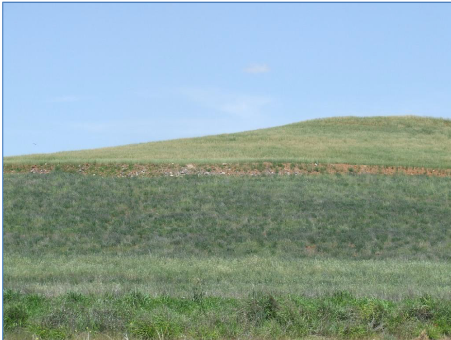
Established cover crop on rehabilitated waste emplacement
